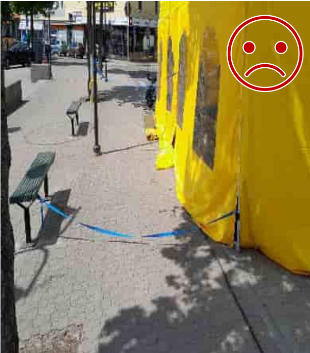
Figure 12 WRONG . Horizontal attachment that does not prevent the tent from rising into the air. Furthermore, the strap is a tripping hazard.
