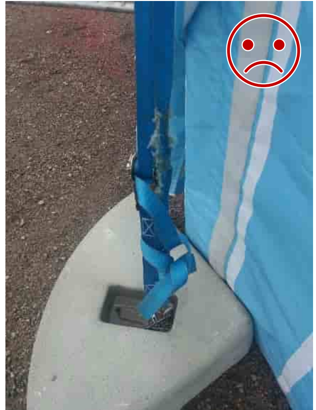
Figure 10 WRONG. The strap is worn.
