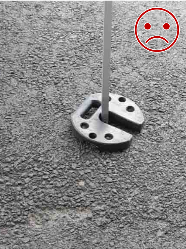
Figure 3 WRONG. The weight is not locked to the structure. It is necessary to have an additional weight on the other side and to lock the weights together.
