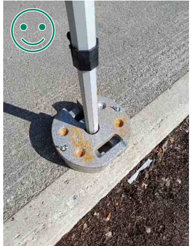
Figure 2 RIGHT. Both weights are secured on both sides with a wing nut. Opposite horseshoe weights prevent the pole from coming loose as the structure shifts. The feet of a corner pole must be able to withstand this weight.
